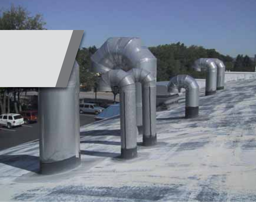
Before: Overview of existing 39-year-old Carlisle roofing system.
