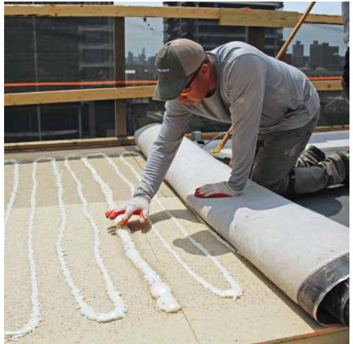
Performing the string time test
