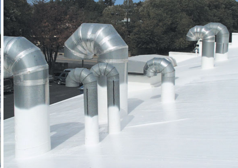
After: Completed restoration.
