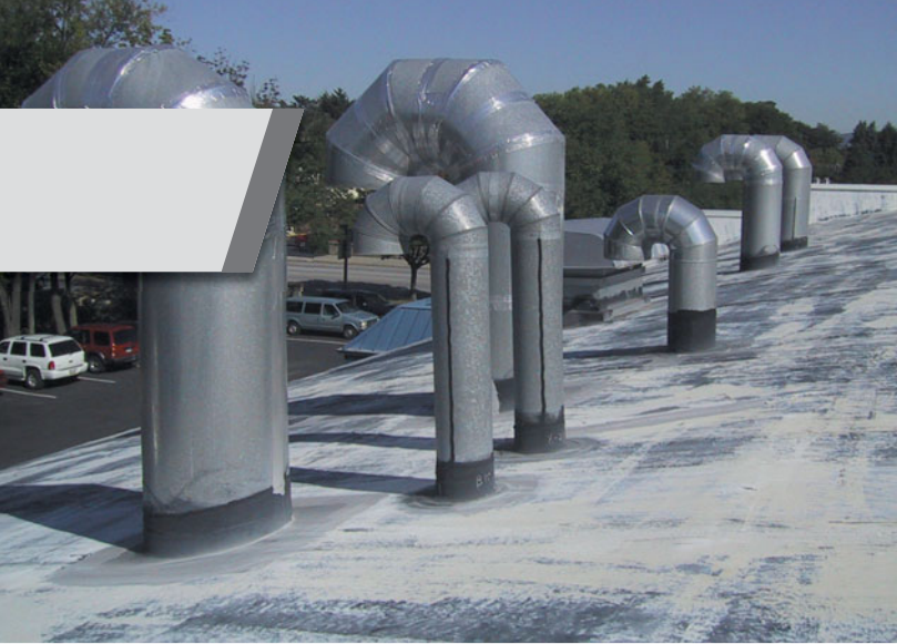
Before: Overview of existing 39-year-old Carlisle roofing system.
